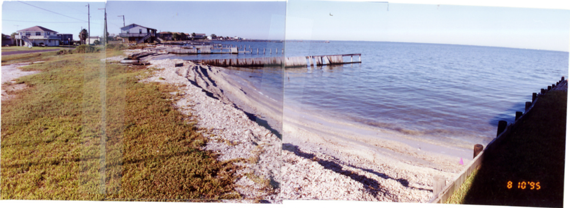
View looking south at Lot 5 in foreground. Lot 6 is in background.
