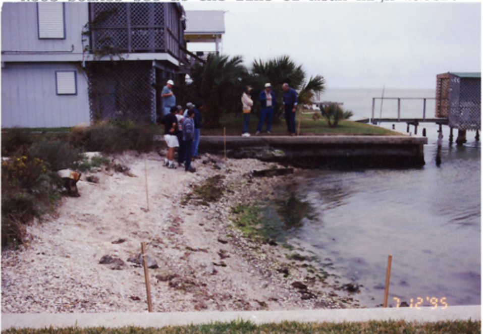
Looking south from north property line at view of shoreline to be bulkhead and filled. Note stakes set at the line of mean high water.
