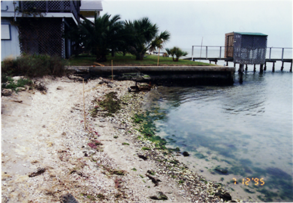
Looking south from northern property line at view of shoreline. Note stakes set at the line of mean high water.
