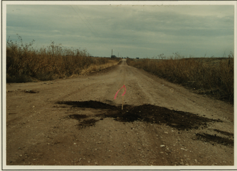
LOOKING NORTH WITH ROAD
