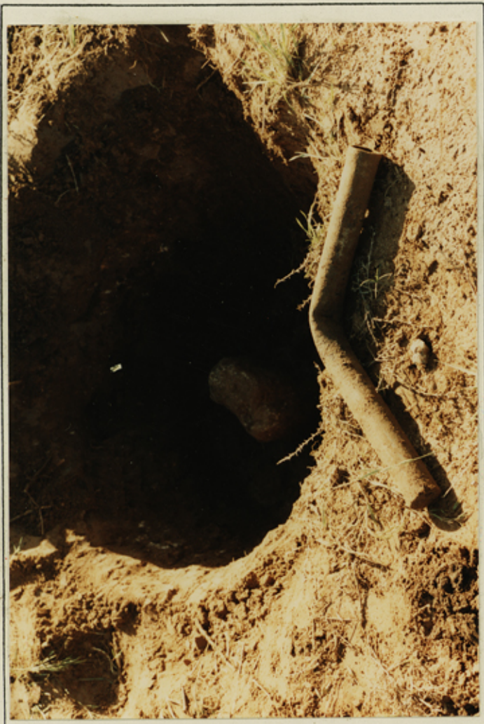
LOOKING EAST (PIPE OUT OF HOLE)
