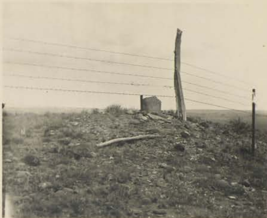
Original Clark Monument No. 16, looking Southeast. One Hundred and Third Meridian.
