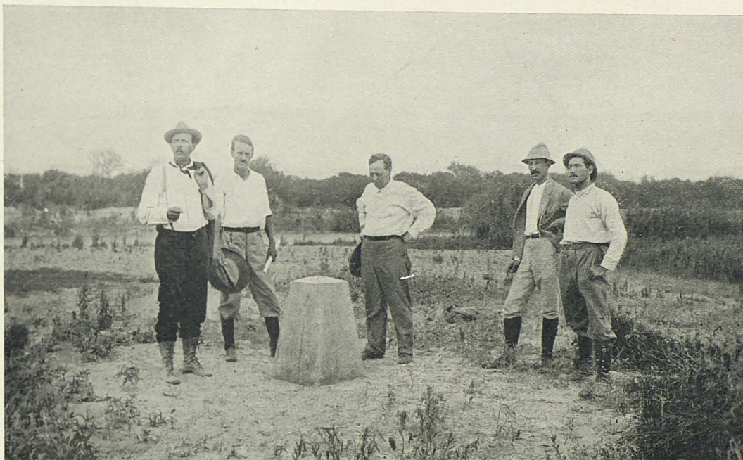
PERMANENT MONUMENT ON "CLOSNER" BANCO NO. 84.
