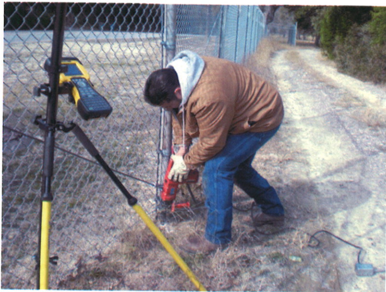
Fig. 10. Mark Hinojosa drilling a hole in concrete at the base of a chain link fence corner post to set a 5/8" iron rod with aluminum cap stamped AGDTX-Boundary. This boundary corner is in the northwest Right-of-Way line of West 35 th Street. View looking northwest.
