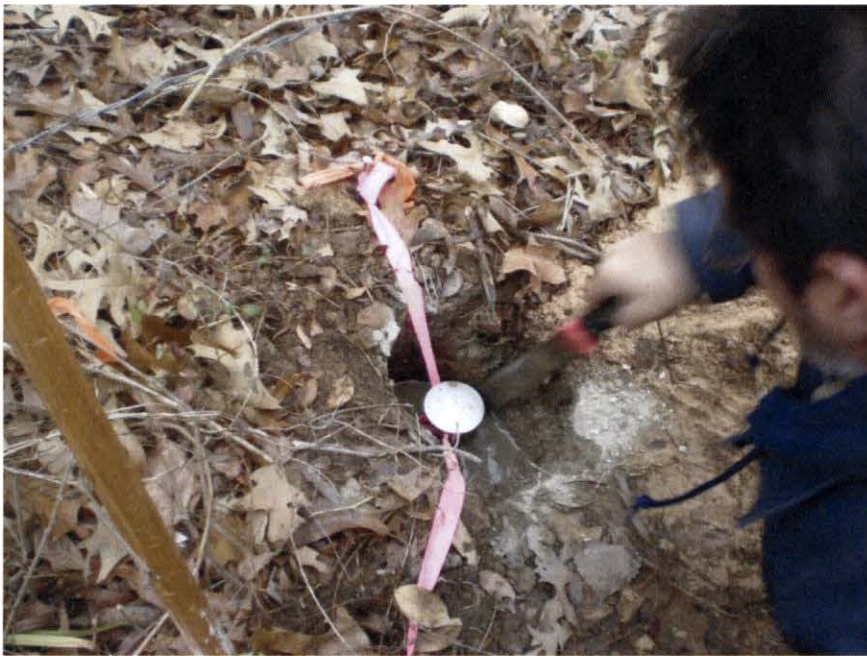
Setting Tract 201 corner at calculated location of lost BC-21 TR 201 (David A. Rolbiecki, RPLS).
