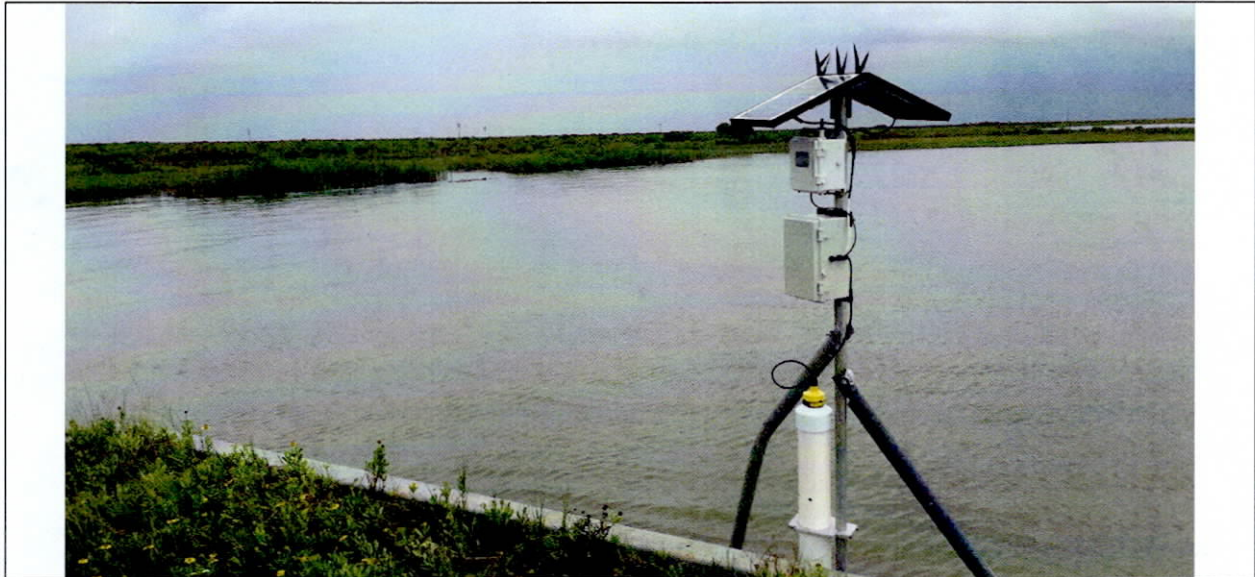
Figure 3: On-site tide gauge setup on Moses Lake
