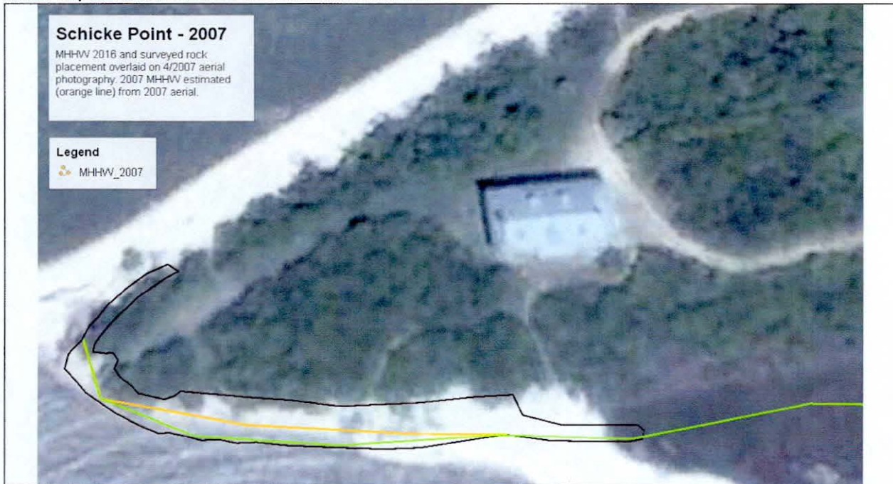
Figure 3: Existing artificial fill exists as a rock revetment along the south shoreline of the west point of Schicke Point. A fill map is shown on sheet 2 of 2 on the map of survey dated AUG 2016.
