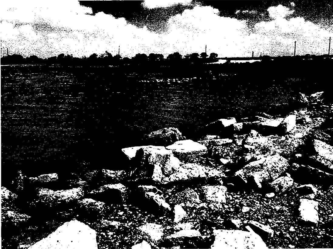
Submerged Jetty, Picture taken from East Jetty
