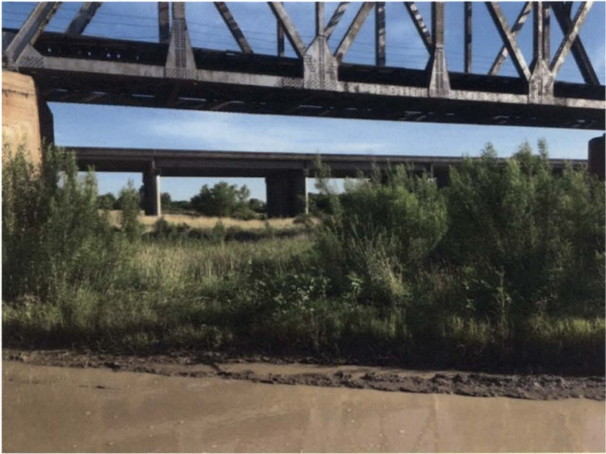
Caption: view looking downstream from railroad crossing toward Hwy 90.
