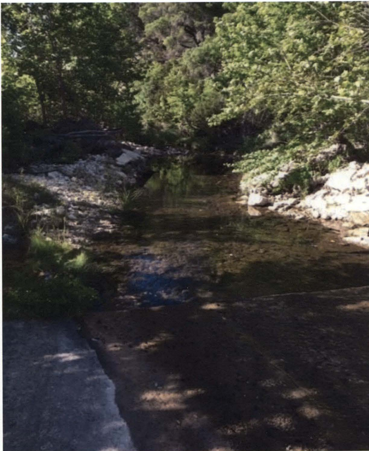
Caption: image of Blanco Creek looking downstream of concrete dam.
