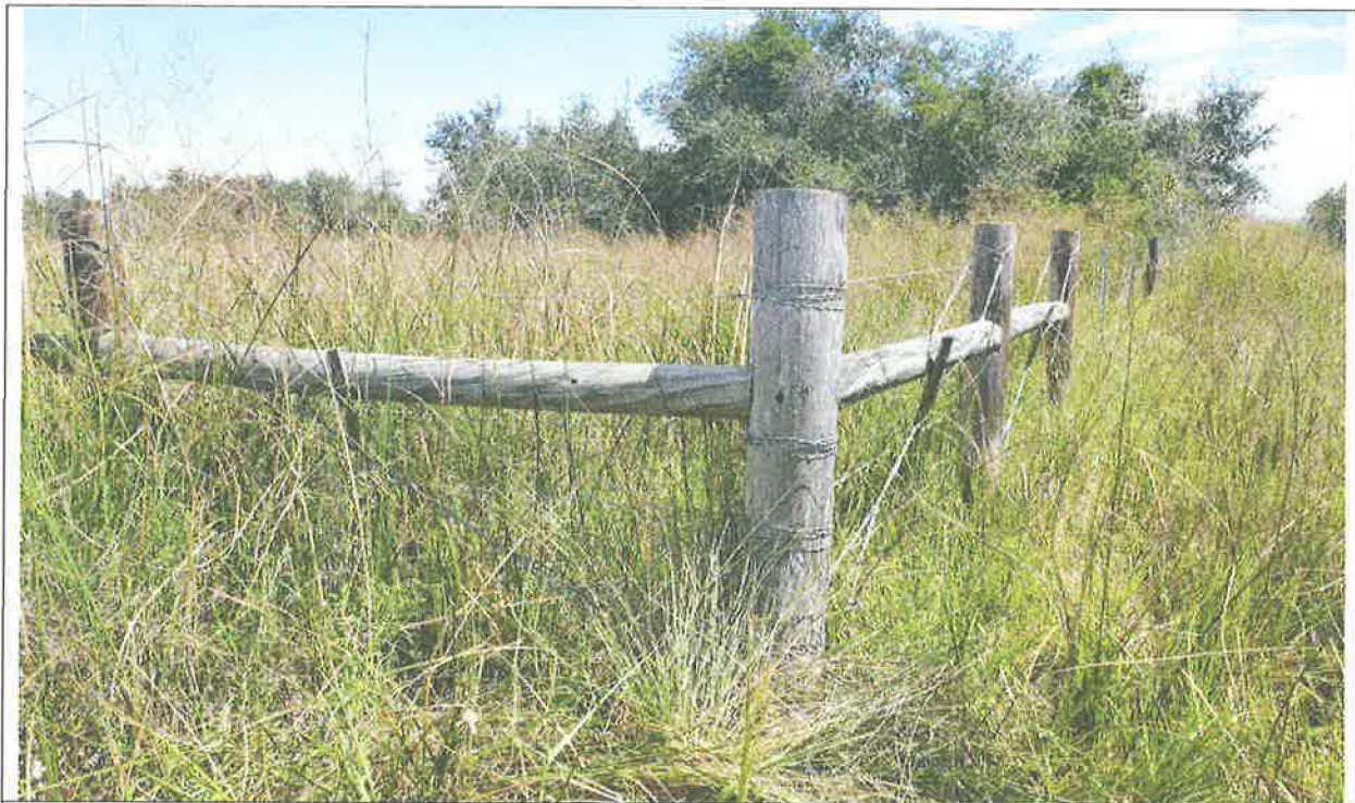
Figure 4: The NORTH end point of the MHW line (littoral boundary) was tied to an apparent refuge corner which was marked with a wooden fence corner post (N:13,303,406.40, E: 2,667,915.38, EL: 12.6')
