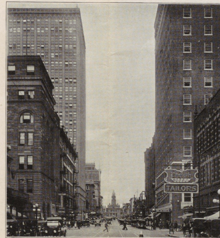
A Street "Canyon" in Fort Worth
