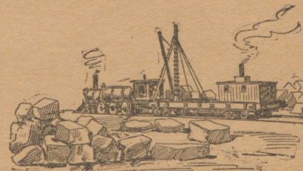
FIVE-TON BLOCKS AND THE MACHINE TO PLACE THEM.
