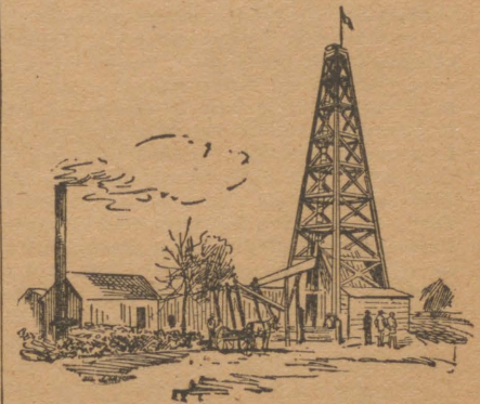
BORING FOR OIL AT BROWNWOOD.
