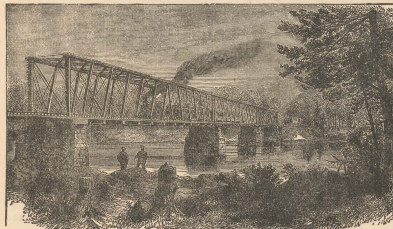
BRIDGE OVER THE SOUTH CANADIAN RIVER ON THE LINE OF THE M., K. & T. RAILWAY.
