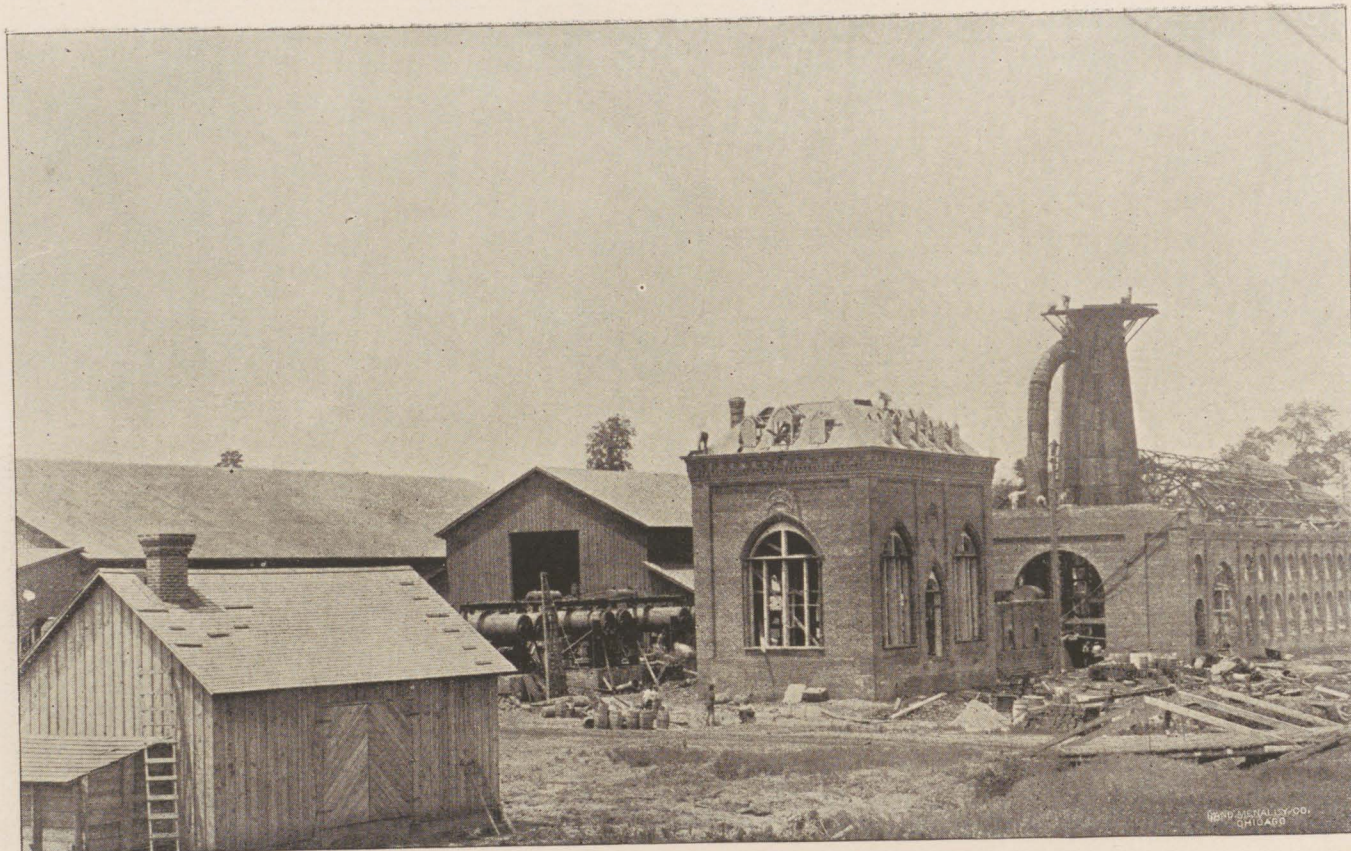
NEW BIRMINGHAM, TEXAS. STAR & CRESCENT IRON FURNACE. Capacity, 50 Tons per Day. Will go into blast in November, '91.
