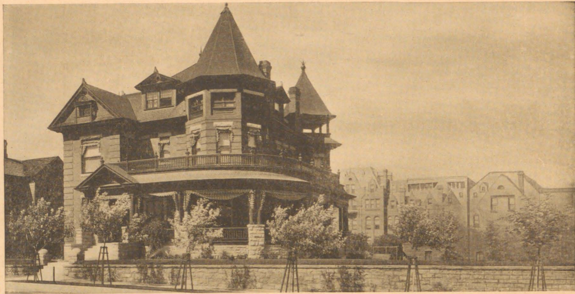
A modern home, El Paso, Texas
