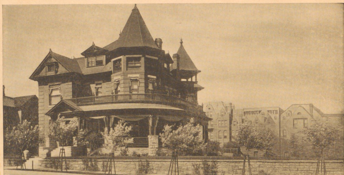
A modern home, El Paso, Texas
