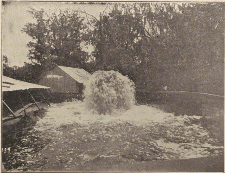
Pumping Plant in Operation.
