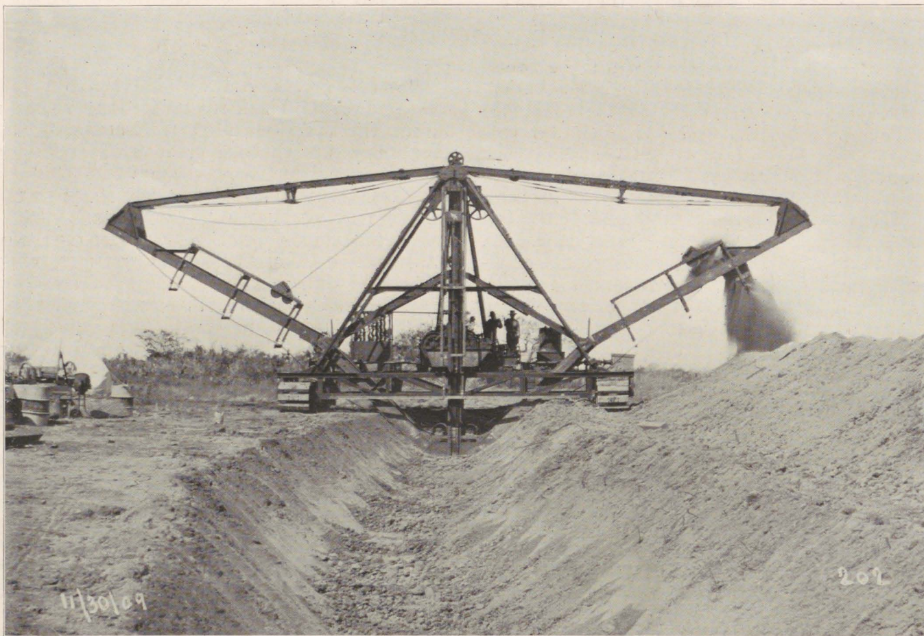
Dredge at Work in the San Benito District.
