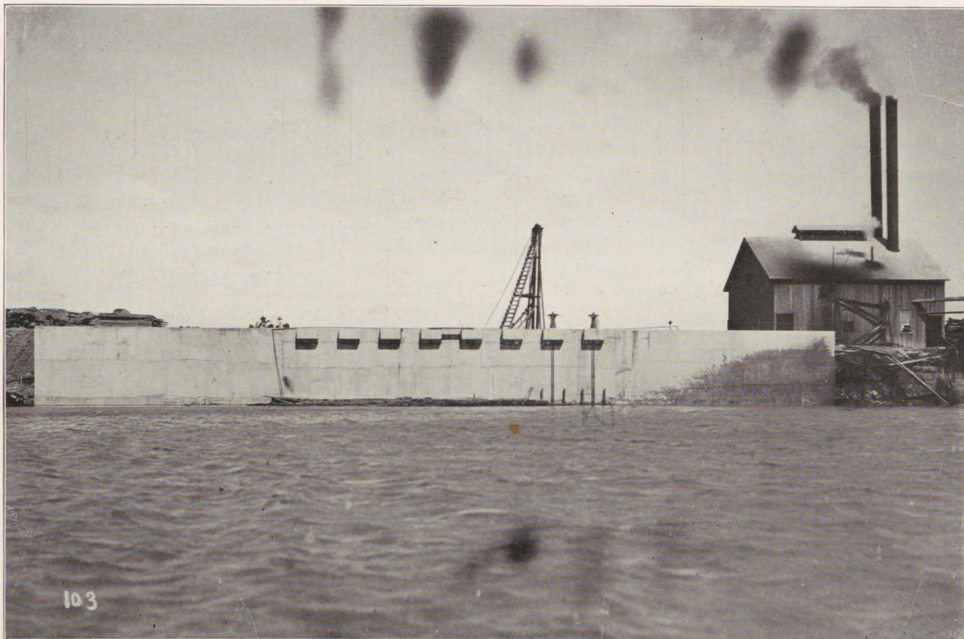
Head Gates of the San Benito Land and Water Company's Main Canal, 225,000 Gallons Capacity Per Minute.
