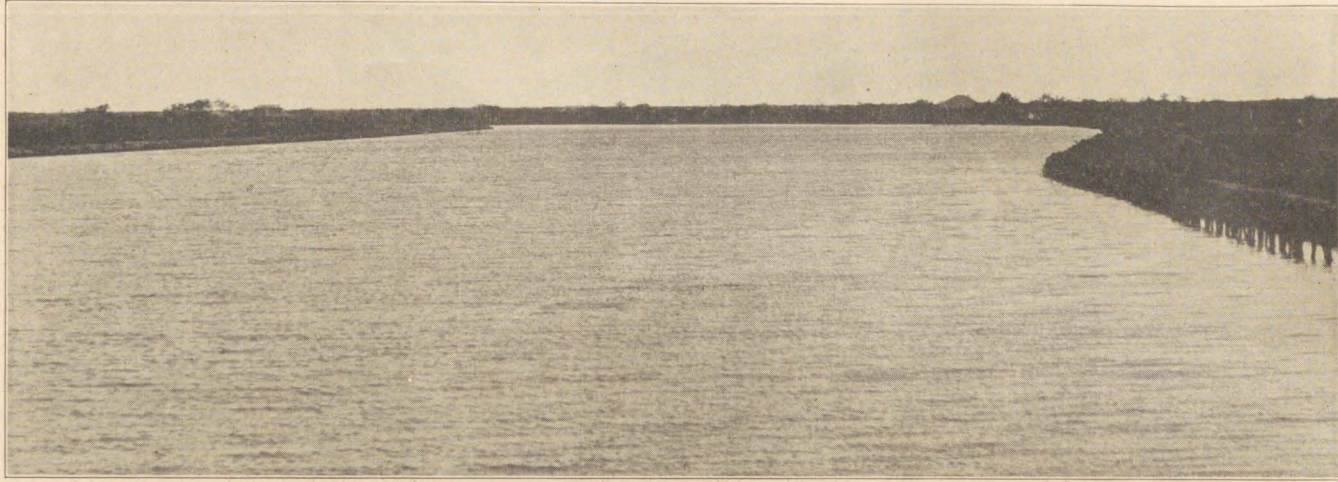
Main Canal at San Benito—37 miles long.
