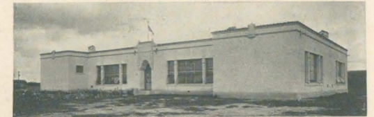
Alamo is in the progressive class with its modern school and new paving program.
