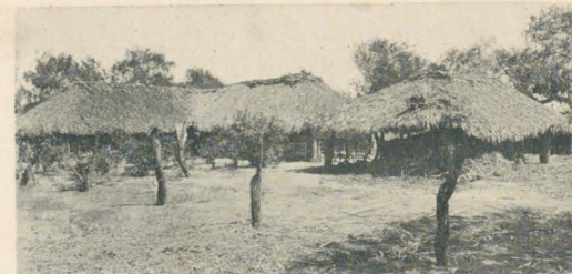
Sector of a typical Mexican jacal village down on Rabb's plantation below Brownsville. The thatch roofs are made of palms from the famous palm grove across the resaca.
