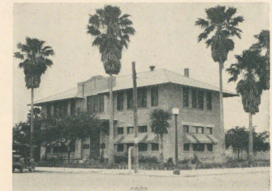
Headquarters of the largest privately owned irrigation system in the world—the American Rio Grande company, of Mercedes.
