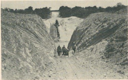
Cutting down through the banks of the Arroyo Colorado to lay the big mains for natural gas supply which is one of the greatest assets the Valley has.
