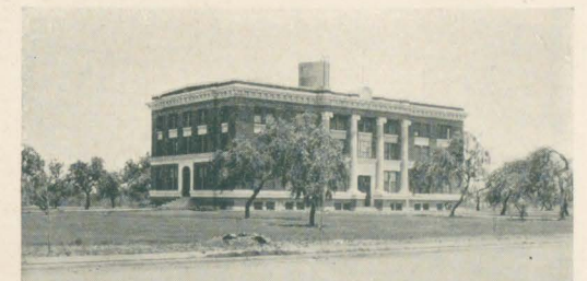
Willacy County court house, at Raymondville which has concrete paved streets from curb to curb.
