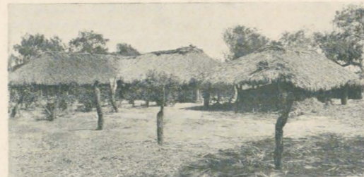
Sector of a typical Mexican jacal village down on Rabb's plantation below Brownsville. The thatch roofs are made of palms from the famous palm grove across the resaca.
