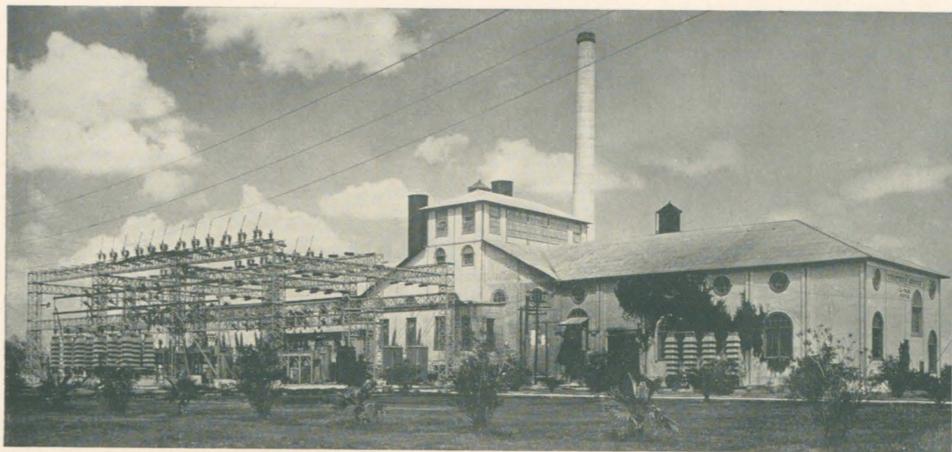
Las Palmas station, San Benito, headquarters of the Valley's electric power supply, consisting at present of twenty-two thousand horse power, distributed over one of the longest transmission lines in the country, more than two hundred and fifty miles, serving more than twenty towns and hundreds of rural homes.
