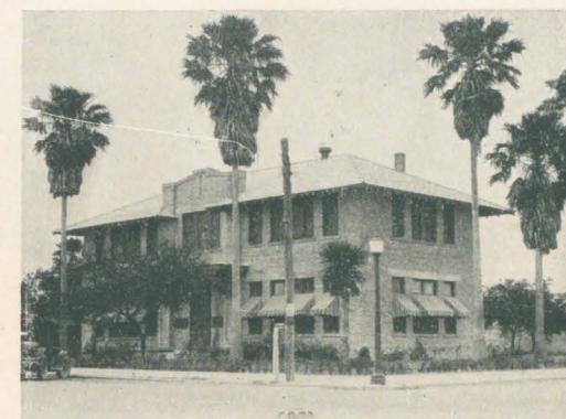
Headquarters of the largest privately owned irrigation system in the world—the American Rio Grande company, of Mercedes.
