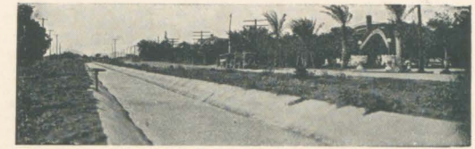
Concrete lined irrigation ditch.
