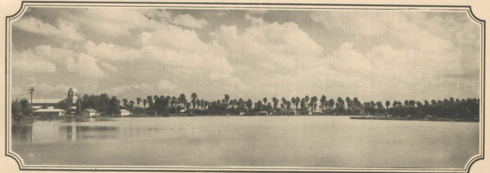
A palm fringed resaca, used as main irrigation canal.
