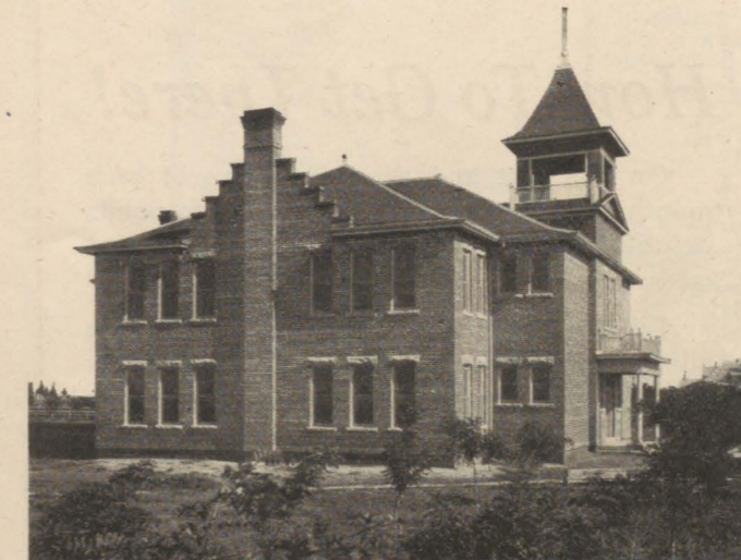
PUBLIC SCHOOL BUILDING, CANYON CITY
