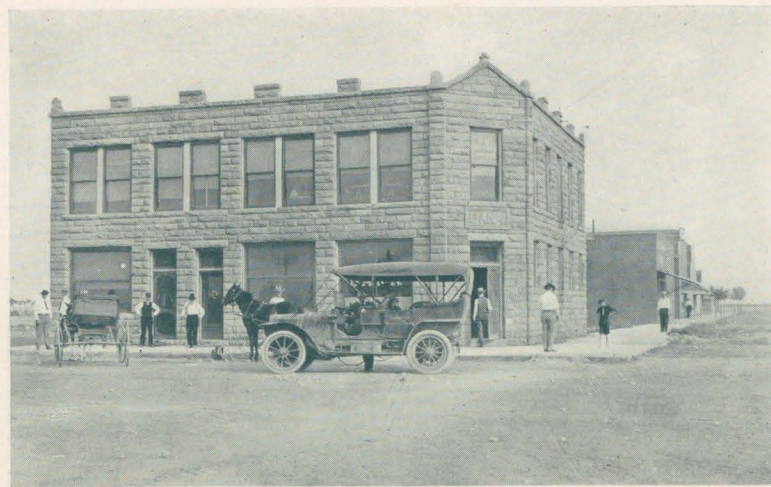
First National Bank Building, Crosbyton. Another concrete block structure.
