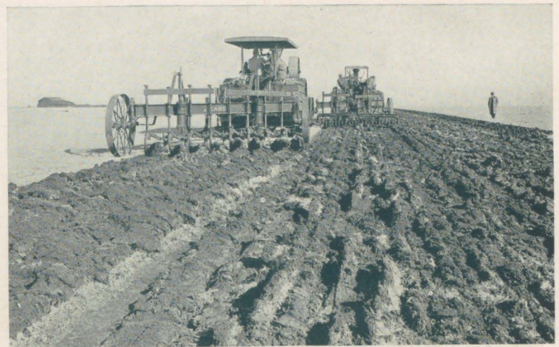
Breaking sod with traction engines. This outfit turns sixteen furrows on every round.
