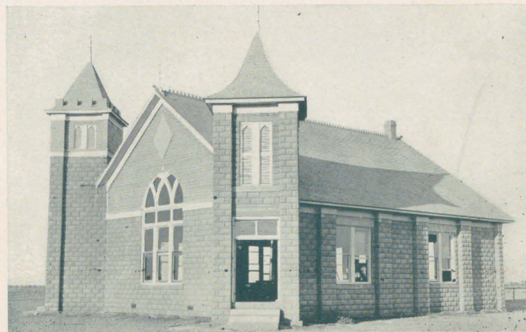
Concrete block church recently erected at Crosbyton, in conformity with plan of uniform improvements.
