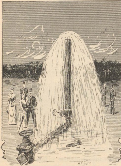
PADGITT'S ARTESIAN WELL, WACO, TEXAS. Supplies 1,400,000 gallons of water a day of 104 degrees Fahrenheit.
