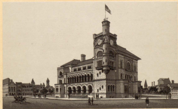
U. S. POST OFFICE AND COURT HOUSE.
