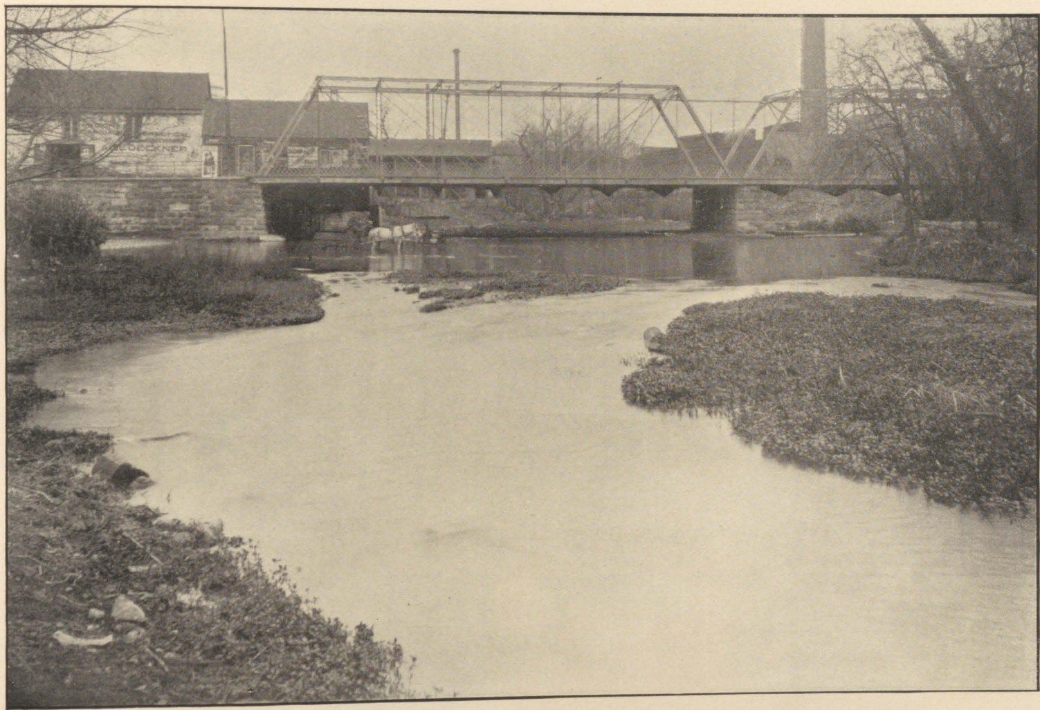
MILL RIVER BRIDGE, SAN ANTONIO RIVER.
