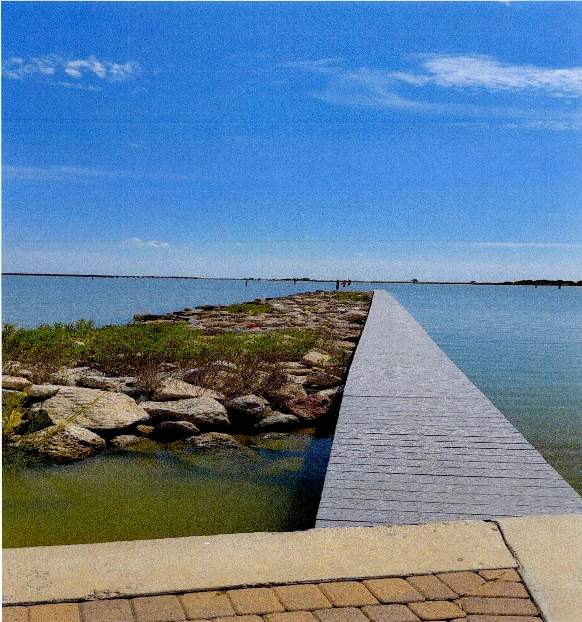
Figure 2: Aransas Bay East Pier, Artificial Fill Area 2 within survey area.
