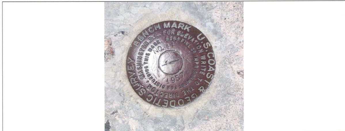
Figure 4: NGS benchmark "877 1510 TIDAL 44" (N: 13,676,511.25, E: 3,310,080.49, EL: 14.45' NAVD88) Shared OPUS Solution
