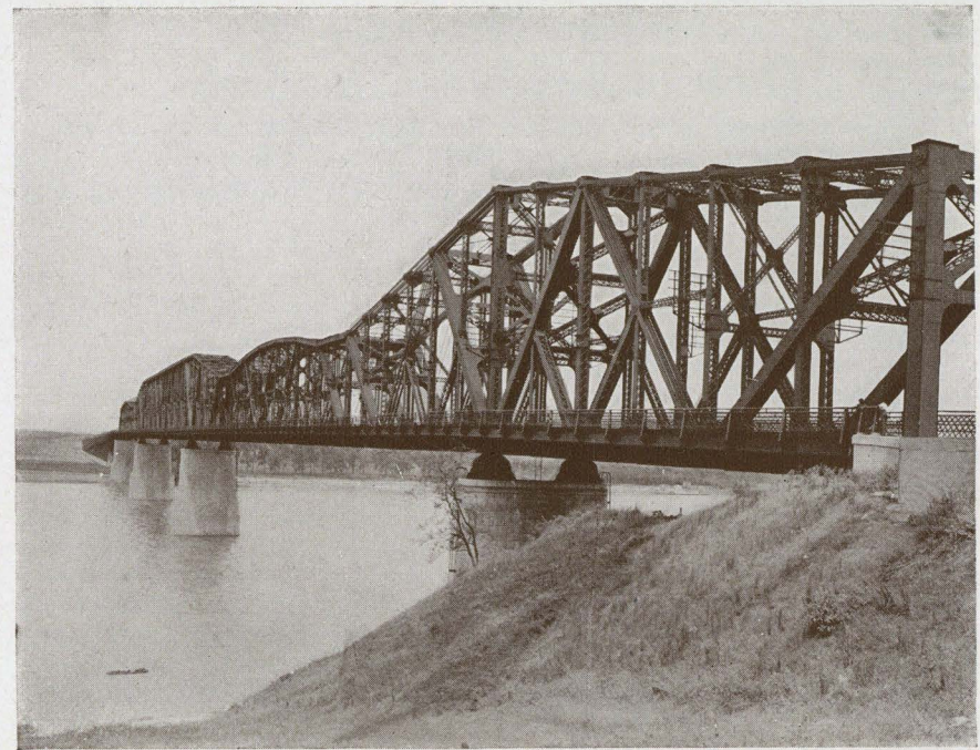
The Missouri Pacific Lines' Bridge Across the Mississippi at Memphis
