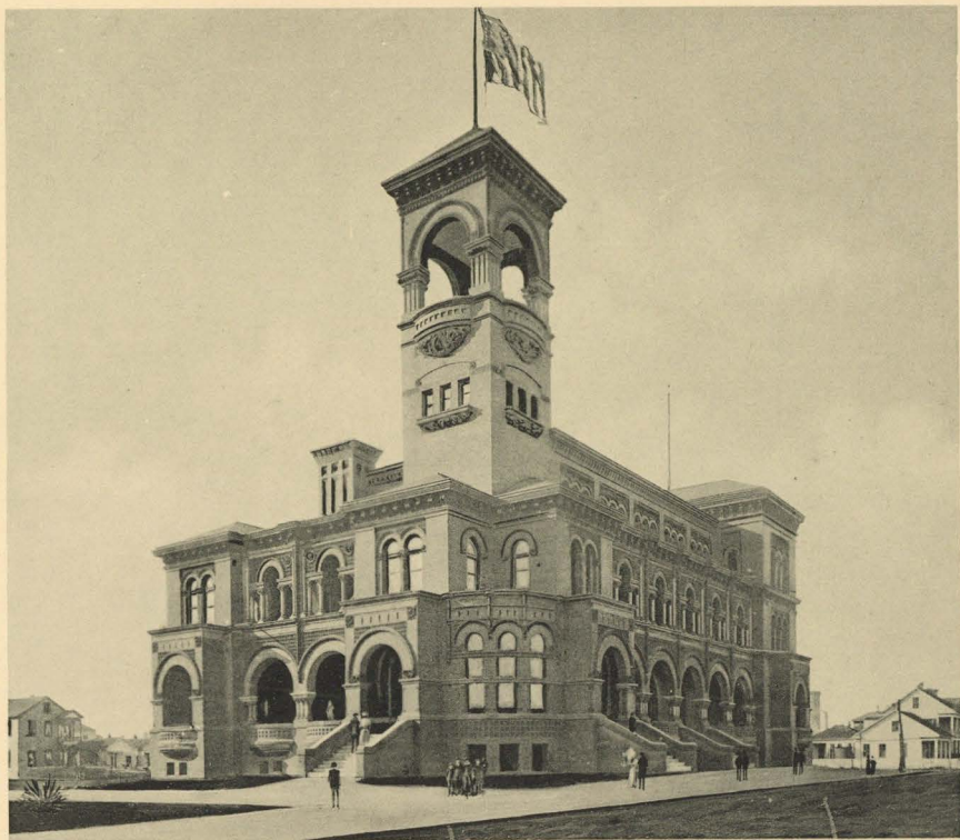
U. S. CUSTOM HOUSE AND POST OFFICE.
