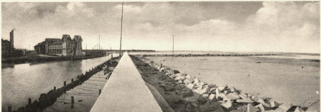
VIEW OF SEA WALL, SOUTH JETTY AND ENTRANCE TO CANAL.
