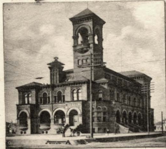
POST OFFICE AND CUSTOM HOUSE.
