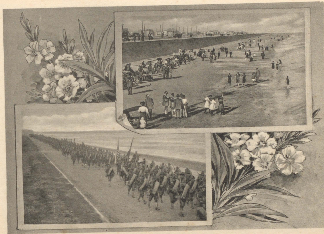
U. S. TROOPS ON SEAWALL BOULEVARD.
