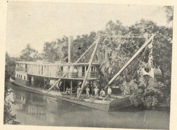
U. S. Dredge Guadalupe at Work on Guadalupe River
