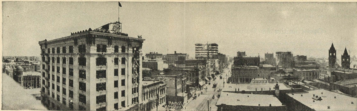
SKYLINE OF HOUSTON, SHOWING MANY NEW BUILDINGS UNDER CONSTRUCTION
