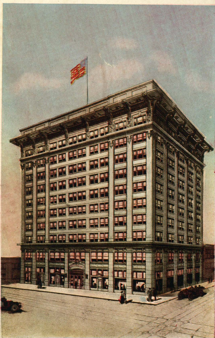
Galveston's First Skyscraper, Said by Experts to Be An Impossibility, Owing to Sandy Nature of Soil. Its Erection Has Proven the Error of This Opinion.
