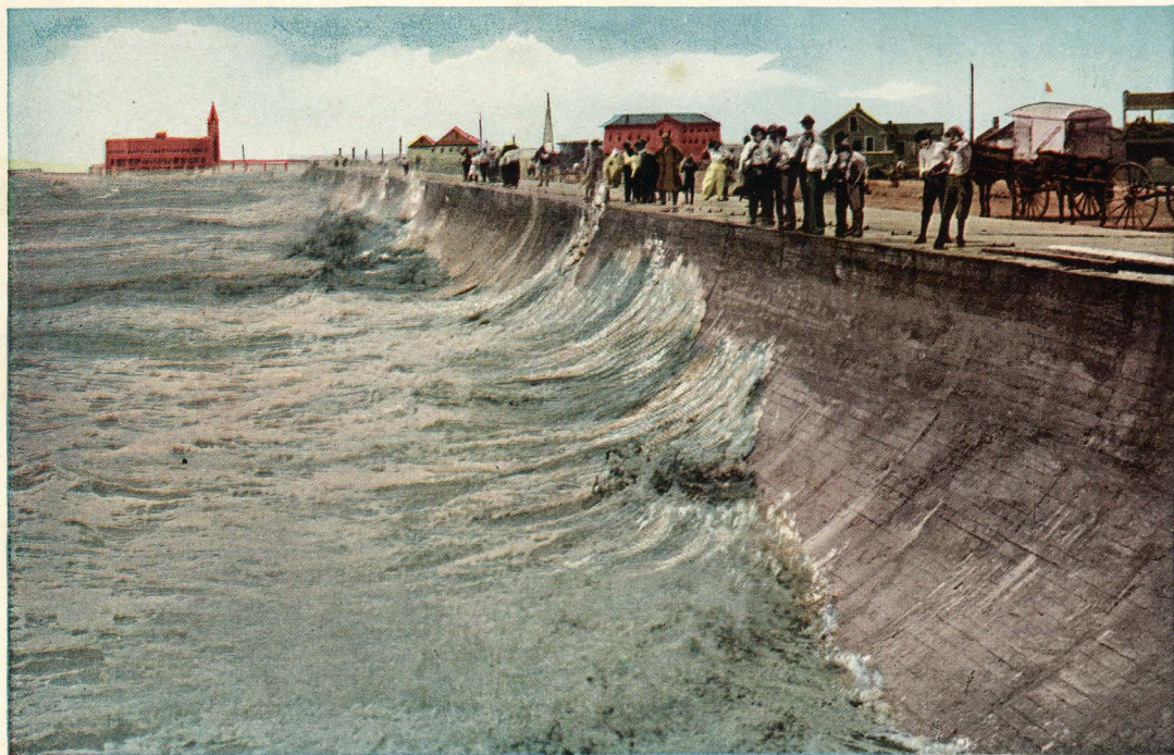
One of the Most Delightful Promenades in the City Is Along the Sea Wall. This Wall Is Five Miles Long and Built of Reinforced Concrete.
