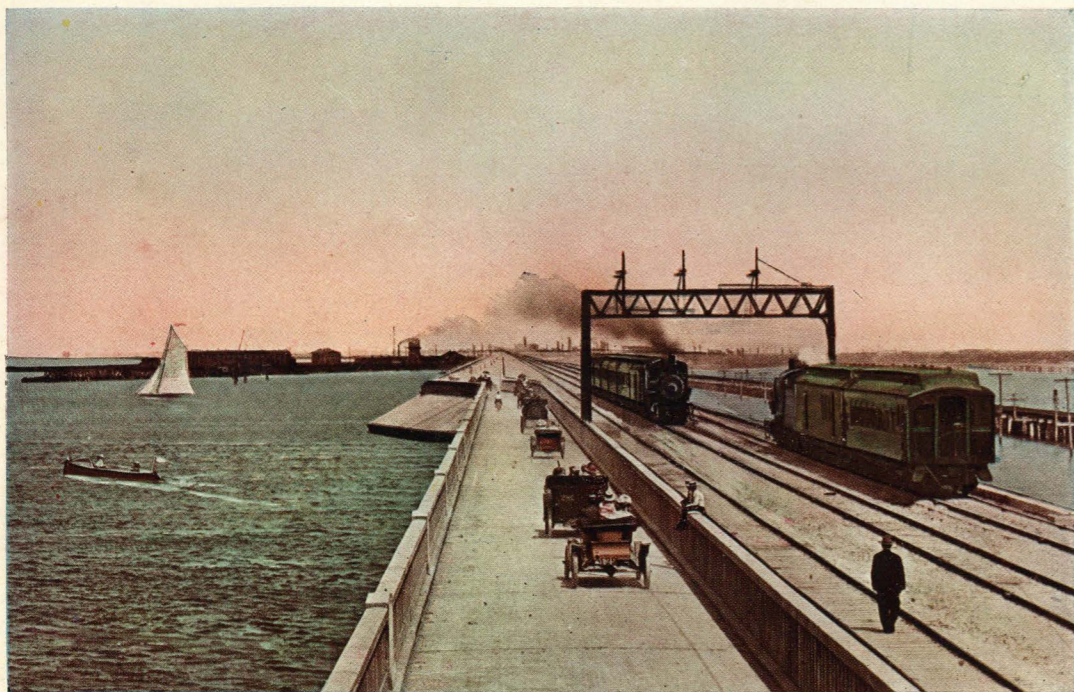
Another View of the Causeway, Showing Old Wooden Trestle Which Has Been Torn Down.
