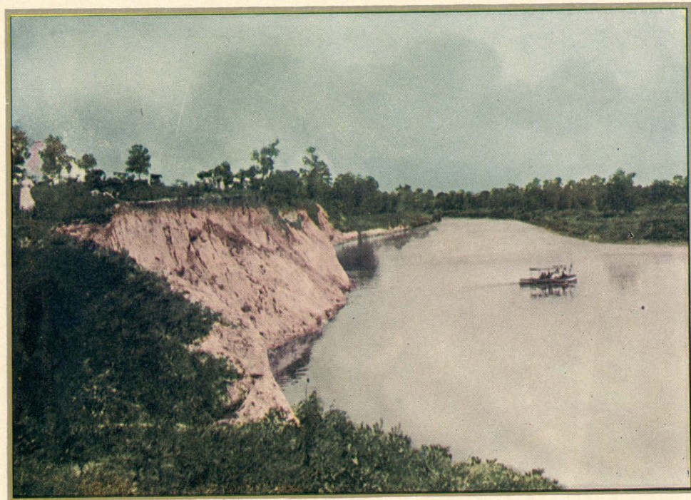
Houston Ship Channel, near Harbor
