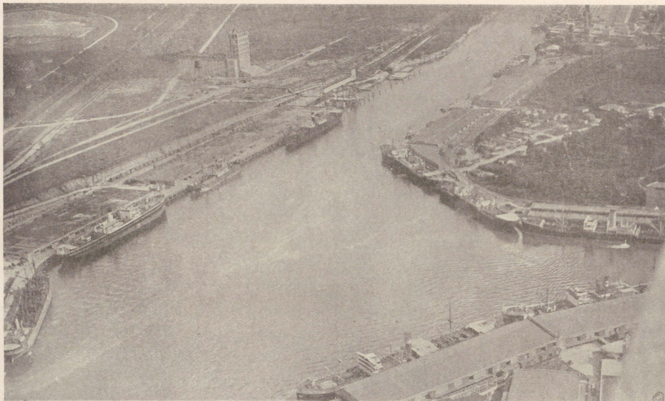
Airview of the Turning Basin Showing Eleven Vessels Loading and Discharging Cargoes
