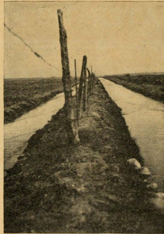
Irrigation Canal Water Running in Two Directions
