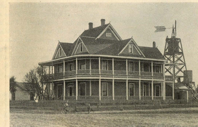
Residence at Toyah, Texas
