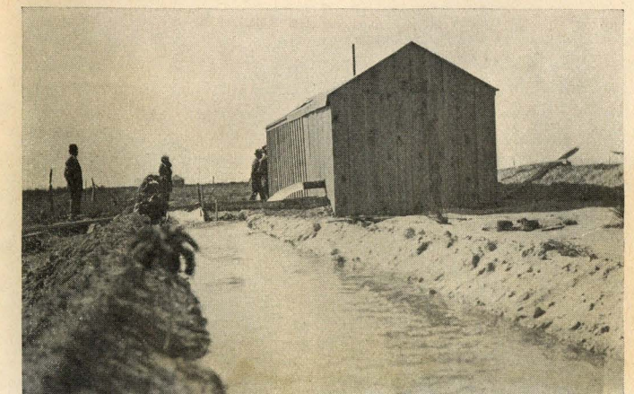
Pumping Plant and Irrigation Canal near Pecos
