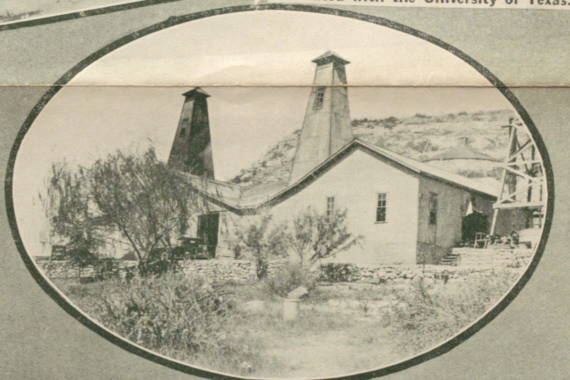
Power Plant and deep wells furnish an abundance of Pure Water.
