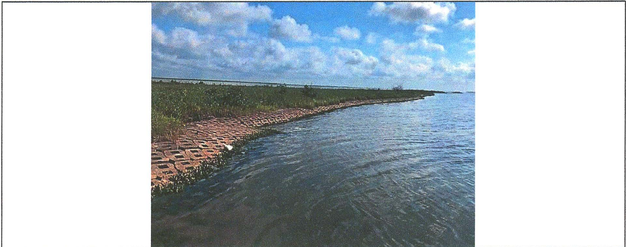
Figure 1: The typical shoreline of Aransas National Wildlife Refuge is covered with concrete matting.
