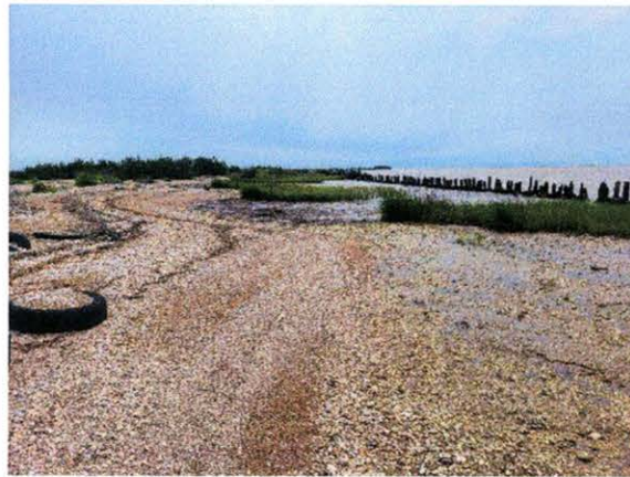
West end of Project showing pilings
