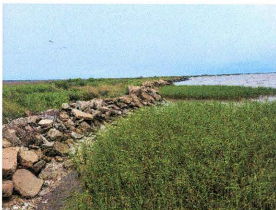
East End of Project showing concrete rip-rap
