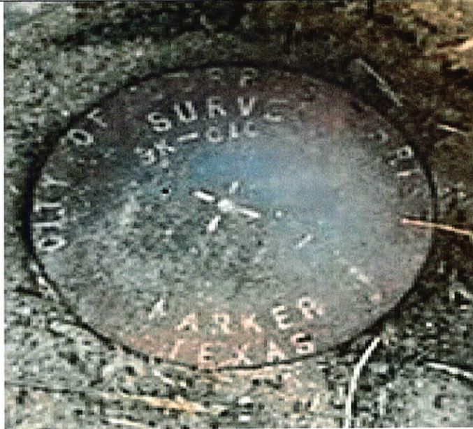
Figure 4: NGS benchmark "AH1675" (N: 17,145,840.83, E: 1,418,646.86, EL: 4.82' NAVD88), Published
